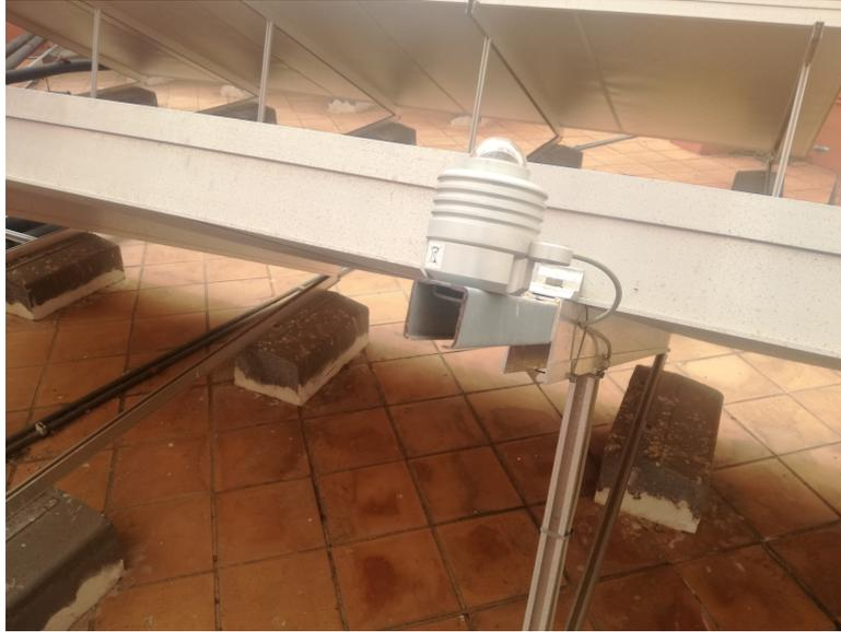
[Figure 13](#): Pyranometer installed in the hotel's rooftop.
