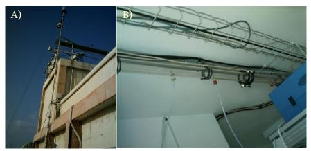
Figure 2.8 A) Design of the sampling inlet line and B) manifold at SCO
