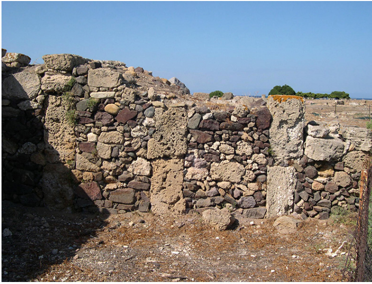
Figure 3. A telaio framework or pillar wall in a house in Nora (Sardinia) (courtesy of F. Prados Martínez).
