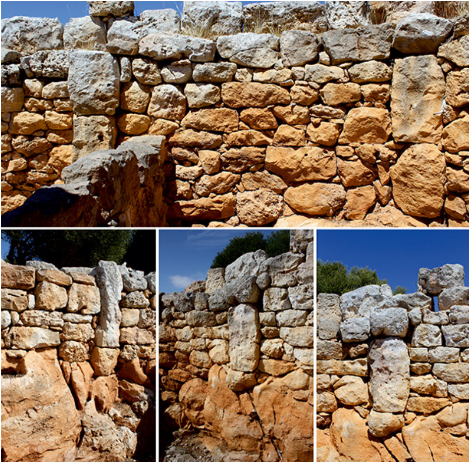
Figure 8. Pillar arrangement in the interior walls of the Torre d'en Galmés dwellings.
