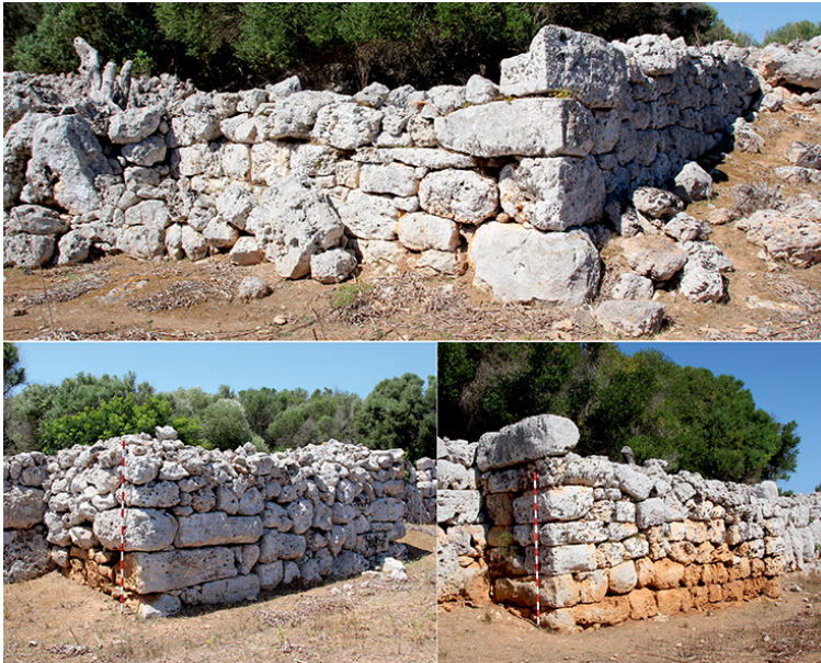
Figure 6. Southeastern corner of the fortified Son Catlar enclosure where cushioned ashlars arranged in alternating headers and stretchers are observed (above); and adjoining bastions that are attached to the east and north of the aforementioned Menorcan town (courtesy of Proyecto Modular).
