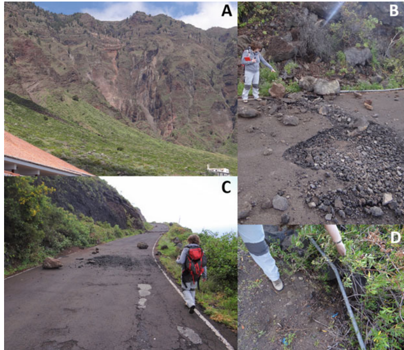
Fig. 12.3 a Las Playas valley scarp. b Rockfalls and impact mark; c Fallen boulders along the road from Tigaday to Sabinosa; d Water pipe bent by a rockfall
