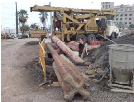
Fig. 3. Drilling machine. Percussion piece, bit.
