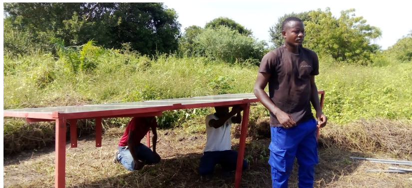
Figure 16: Installation of solar panels
