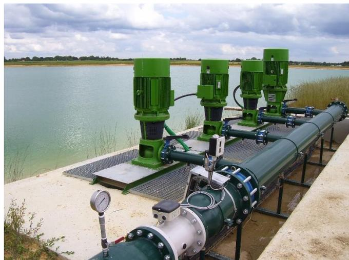
**Figura 9: Bombas centrífugas verticales (Rovatti Pompe)**
