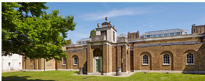
Figura 35. La Dulwich Picture Gallery. https://www.dulwichpicturegallery.org.uk/planning-your-visit/gardens/
