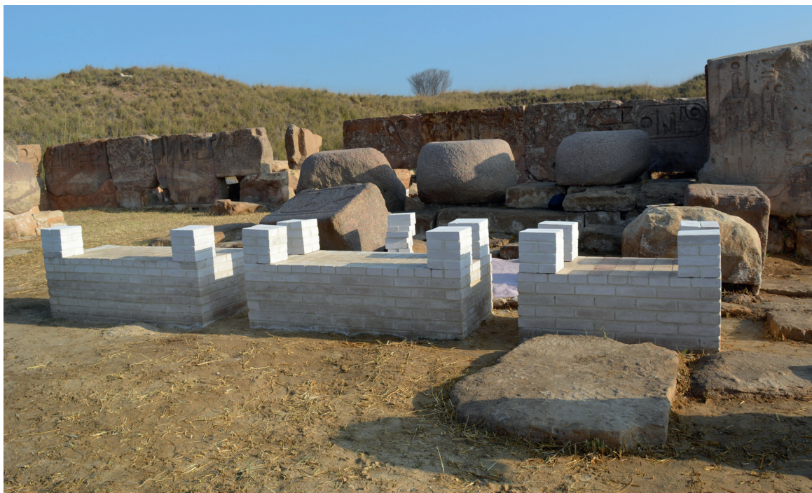
Figure 30. Pedestals prepared for architraves.
