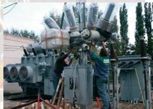
Fig.2 The stand and control panel are fixed in place.
