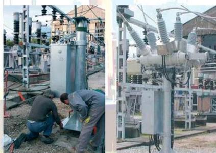
Fig. 3 The module is assembled on the stand.
