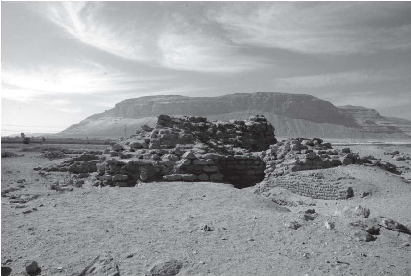
Figure 3. The pyramid of Sinki, near Abydos. This monument was left unfinished. Notice the mud-brick construction ramps still attached to the sides of the pyramid.
