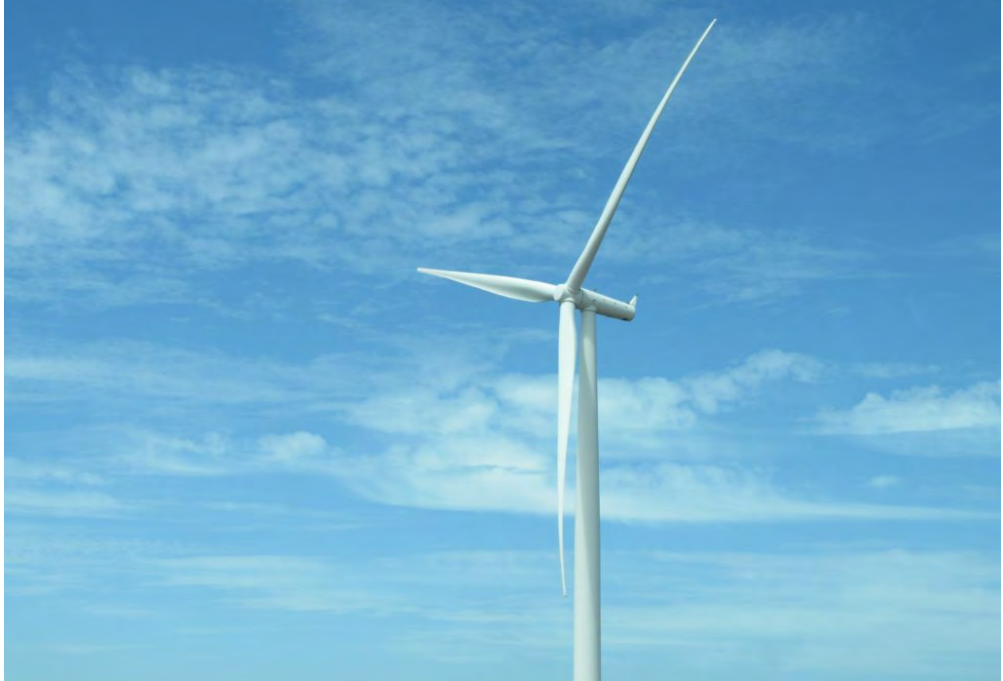
Figure 4.29: An image of a horizontal axis wind turbine 8
