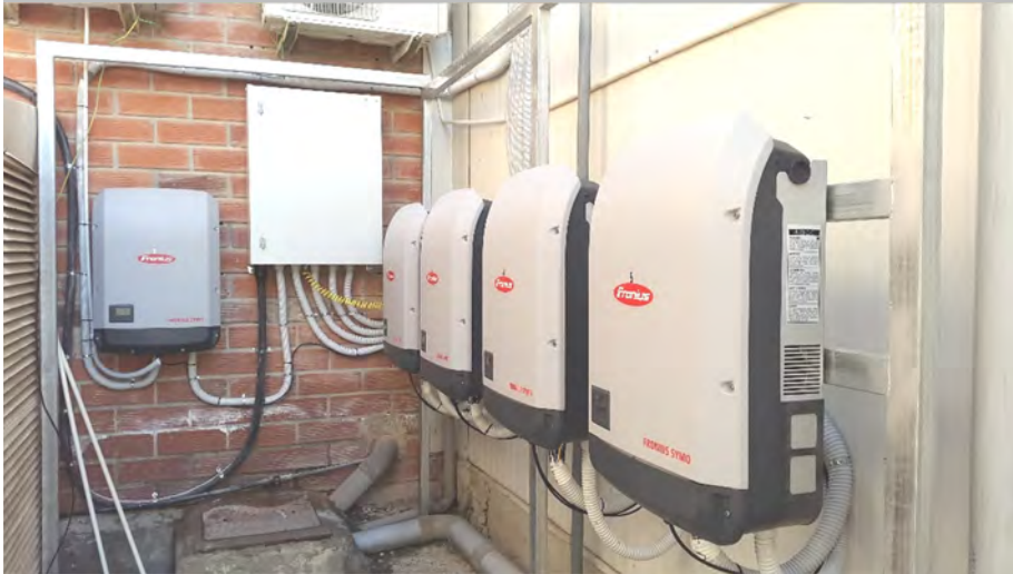
Figure 4.21: Inverter installation with switchgear
