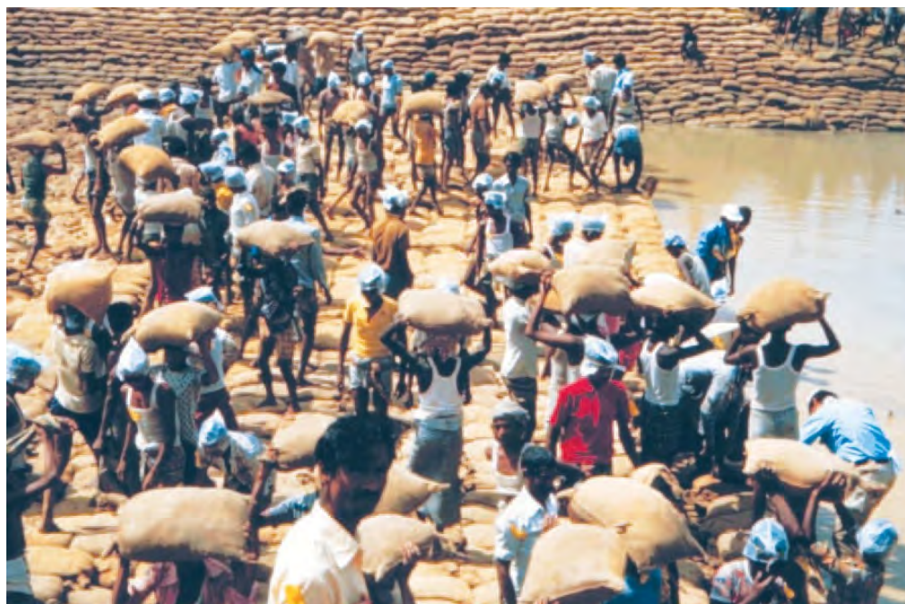
Figure 1.25: Closure dam under construction at Jamuna river, Bangladesh
