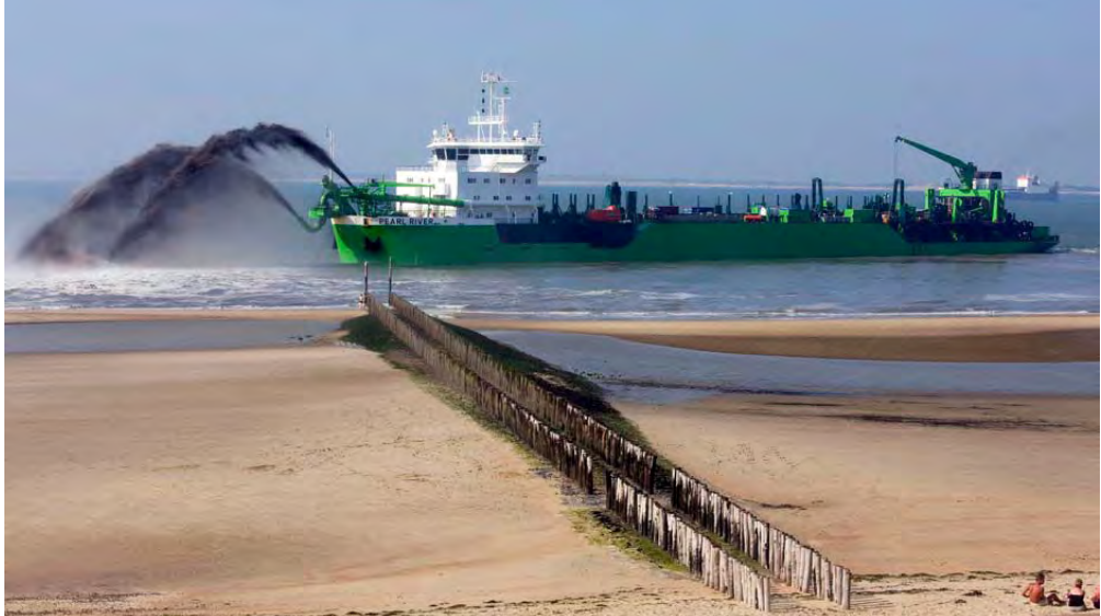
Figure 1.11. The rainbow method of transferring nutrients to the shore Slurry is discharged via a jet at the bow of the ship once it has been sailed as close to the shore as possible
