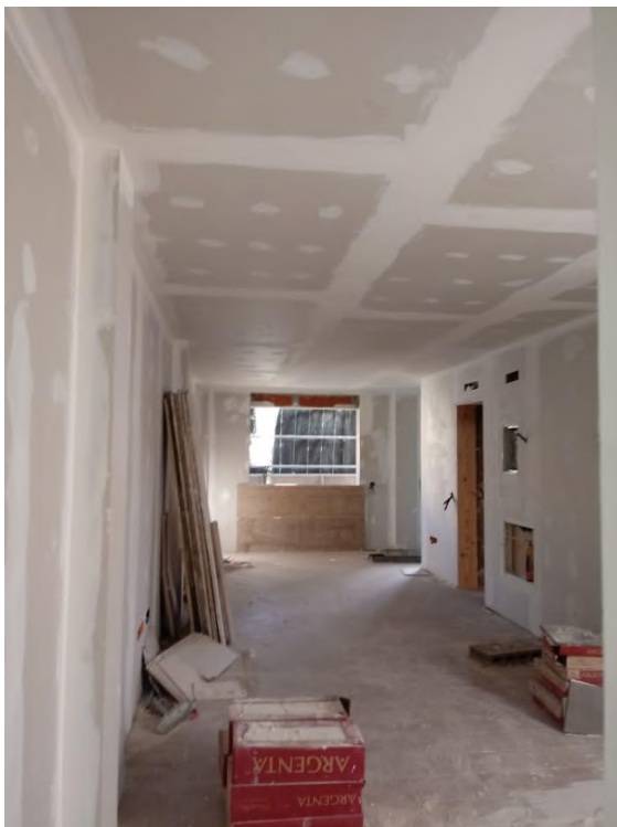
Fig 36 Falso techo continuo
