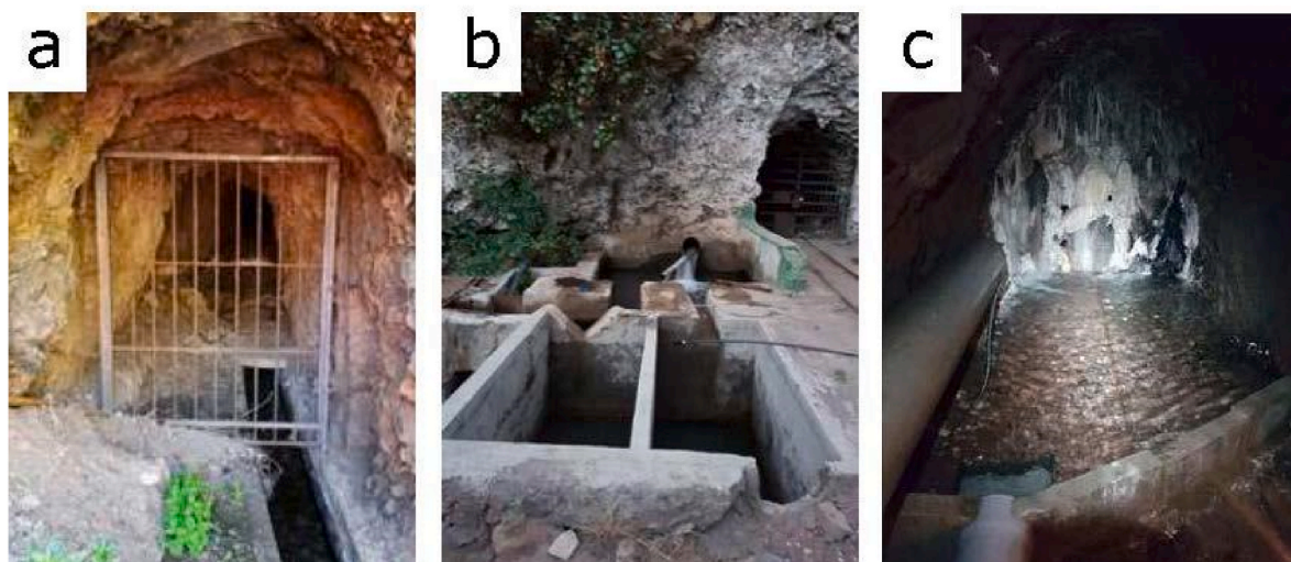
Fig. 1. Groundwater tunnel a) the tunnel mouth, b) water collection c) tunnel end.
